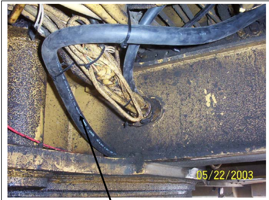
Hose and wiring at cab side of bulkhead wall.
