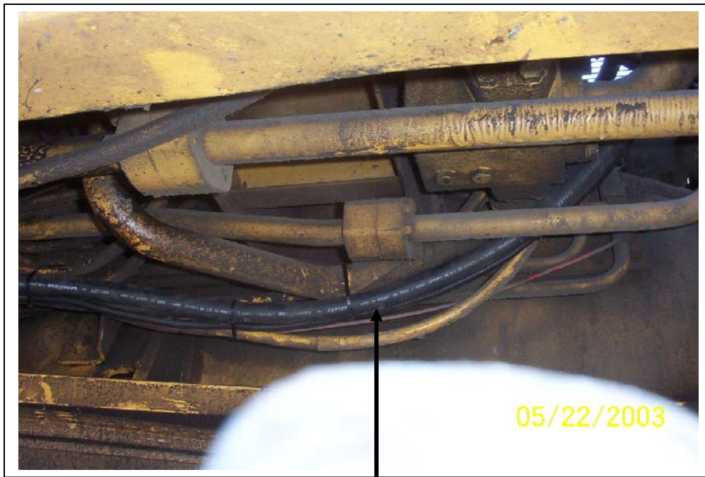
Hose and wiring running up towards the cab.
